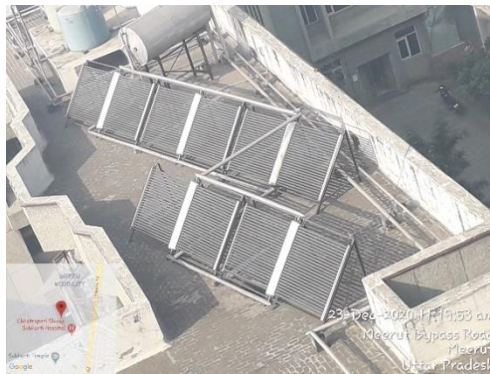
13. 02 Solar Water Heater of capacity 2,500 LPD each installed in Hardyal Singh (Couple Accommodation)
