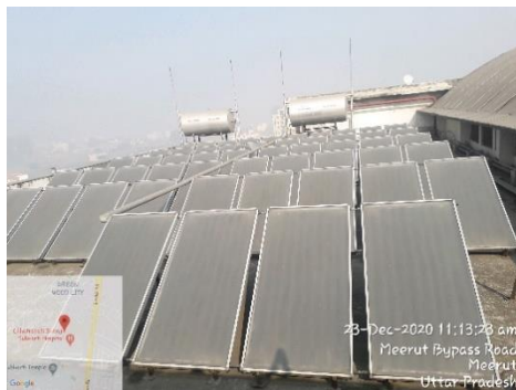
11. 02 Solar Water Heater of capacity 2,500 LPD each installed in Lachit Boys Hostel
