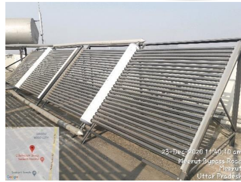
12. 02 Solar Water Heater of capacity 2,500 LPD each installed in Udham Singh Boys Hostel.
