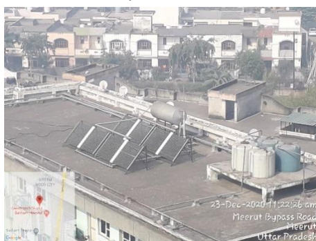
13. 02 Solar Water Heater of capacity 2,500 LPD each installed in Hardyal Singh (Couple Accommodation)
