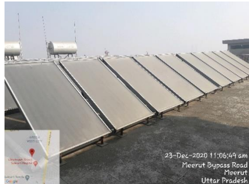
10. 09 Solar Water Heater of capacity 2,500 LPD each installed in Gohin, Shyam Krishna & Kotnish Boys Hostels.
