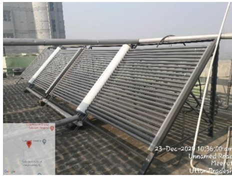
10. 09 Solar Water Heater of capacity 2,500 LPD each installed in Gohin, Shyam Krishna & Kotnish Boys Hostels.
