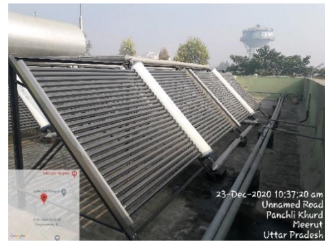
10. 09 Solar Water Heater of capacity 2,500 LPD each installed in Gohin, Shyam Krishna & Kotnish Boys Hostels.
