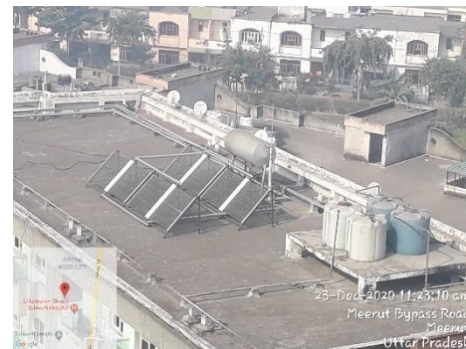
13. 02 Solar Water Heater of capacity 2,500 LPD each installed in Hardyal Singh (Couple Accommodation)
