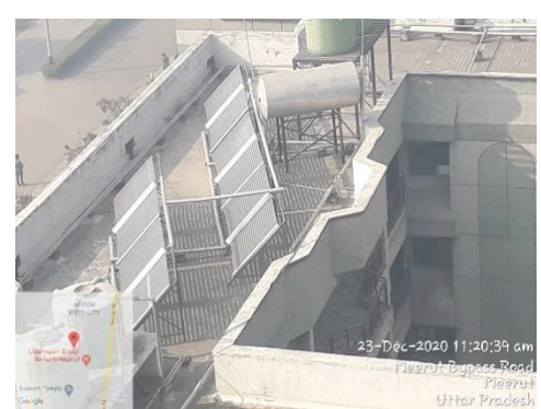
13. 02 Solar Water Heater of capacity 2,500 LPD each installed in Hardyal Singh (Couple Accommodation)
