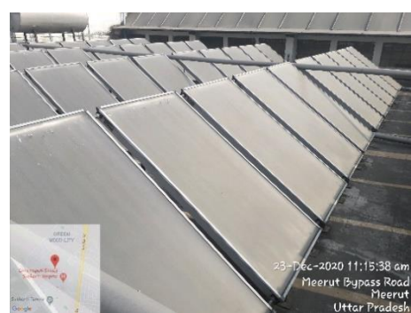
11. 02 Solar Water Heater of capacity 2,500 LPD each installed in Lachit Boys Hostel
