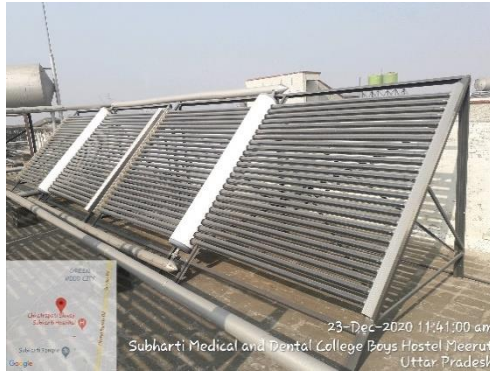
12. 02 Solar Water Heater of capacity 2,500 LPD each installed in Udham Singh Boys Hostel.
