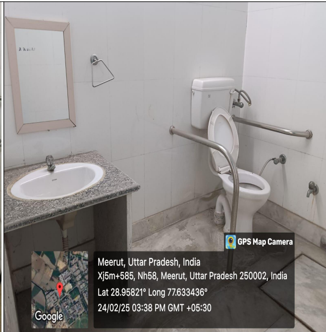
WASHROOM IN MLD BOYS HOSEL
