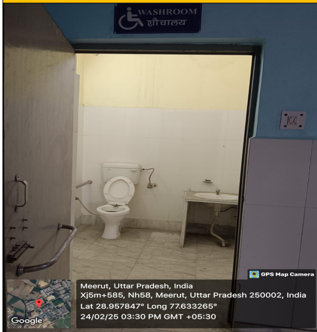
WASHROOM IN AD BOYS HOSTEL
