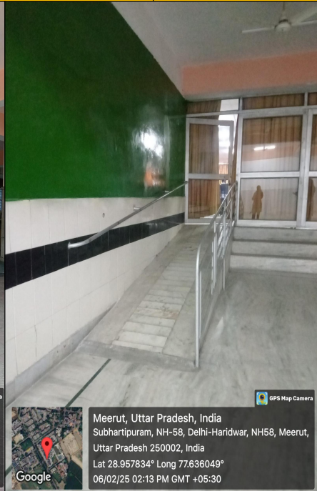
RAMP AT THE ENTRANCE OF COUNCIL HALL
