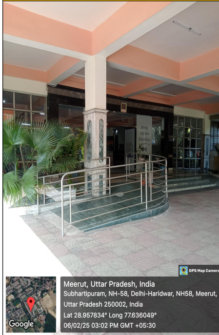
RAMP AT MAIN ENTRANCE GATE
