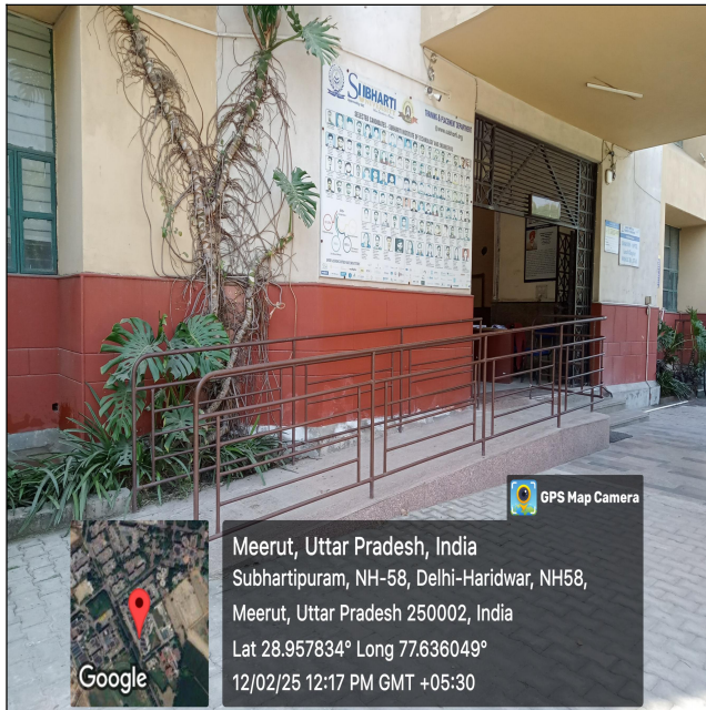
RAMPS AT ENTRANCE GATE
