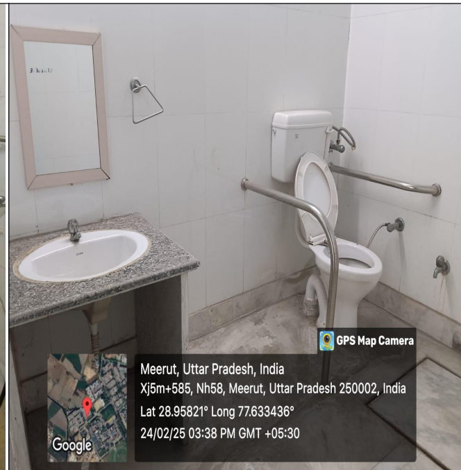
WASHROOM IN MLD BOYS HOSEL
