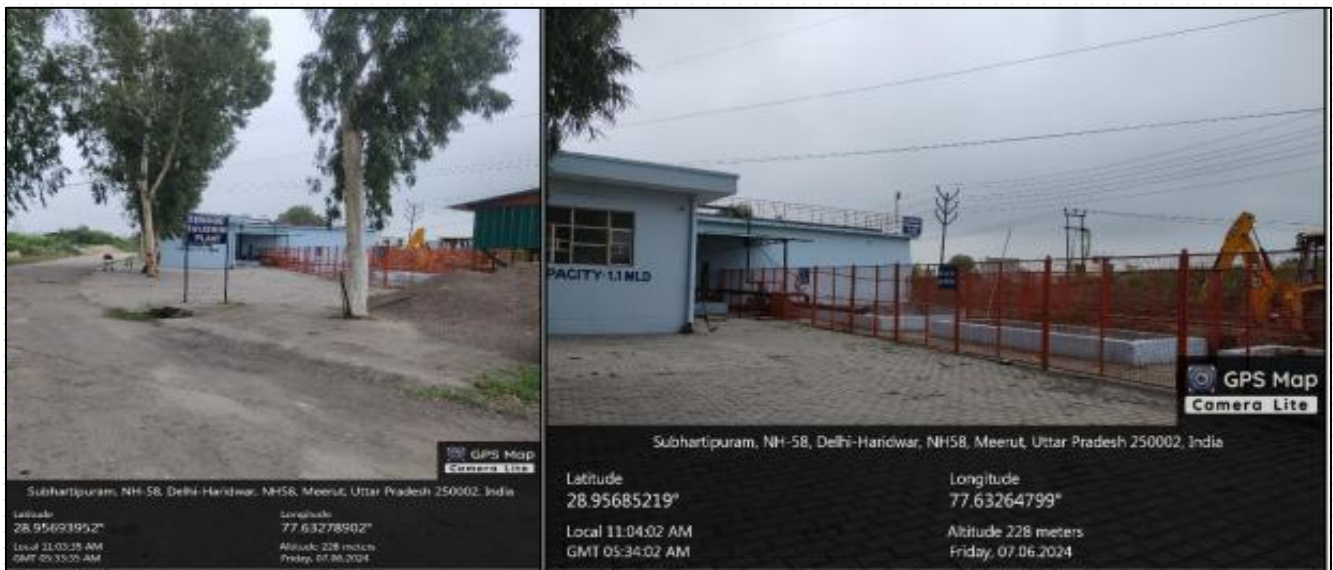
Waste Water Recycling
